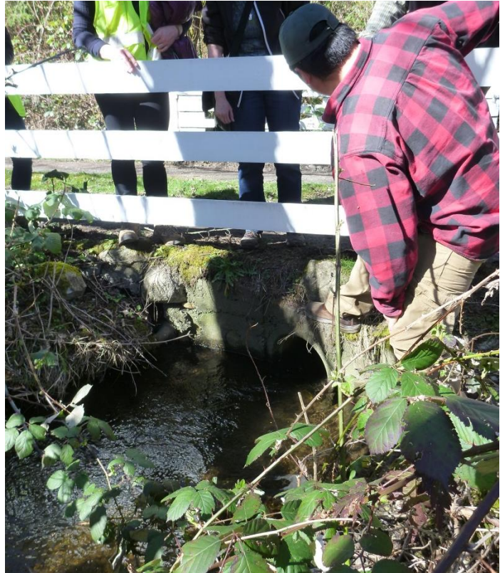
Figure 3. Undersized culvert C6.
