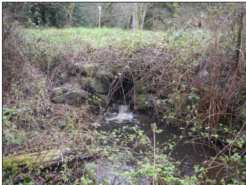
Figure 2. Looking North towards High School Road and perched culvert (C1) outflow into 580-ft ditch.
