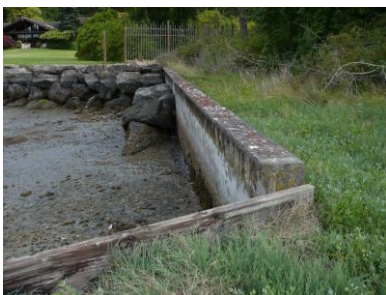
Examples of existing armor on the Powel property. Under the restoration design, the armor in these areas would be removed.
