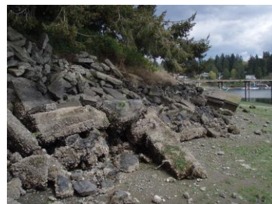
Examples of existing armor on the Powel property. Under the restoration design, the armor in these areas would be removed.
