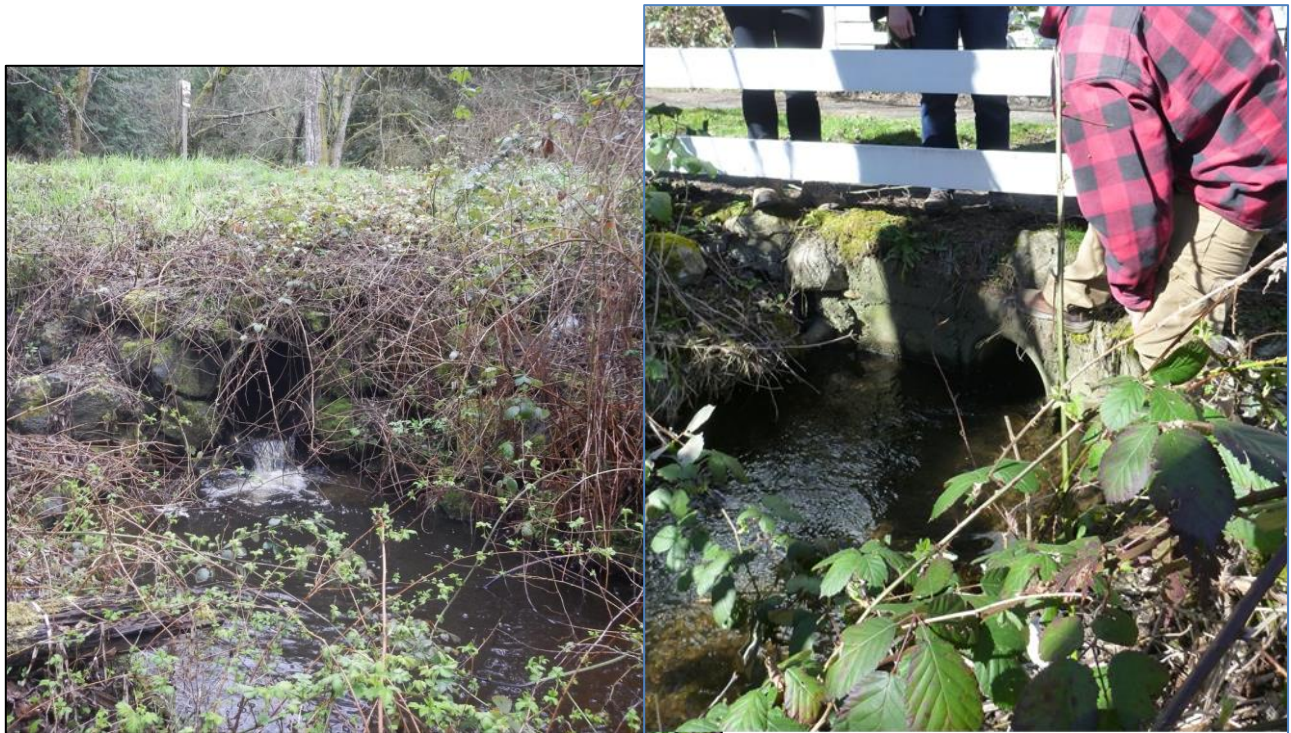
Figure 35. High School Road perched culvert C1 and undersized culvert C6.
